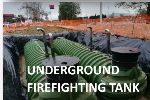
UNDERGROUND FIREFIGHTING TANK
