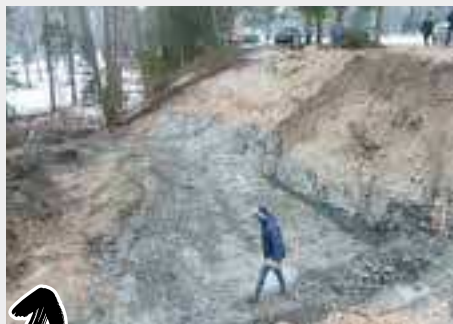
Visit the construction site
